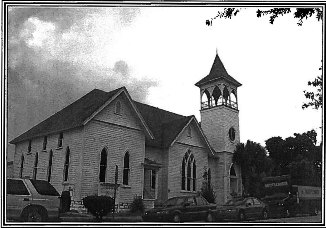
Photo 2 View from Northwest
